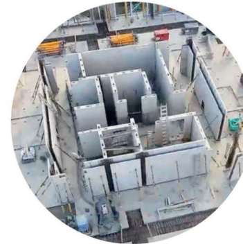
Pre-cast concrete shear / core walls
